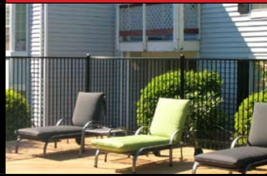
5' 2-Rail Ornamental Iron - Pool Fence
